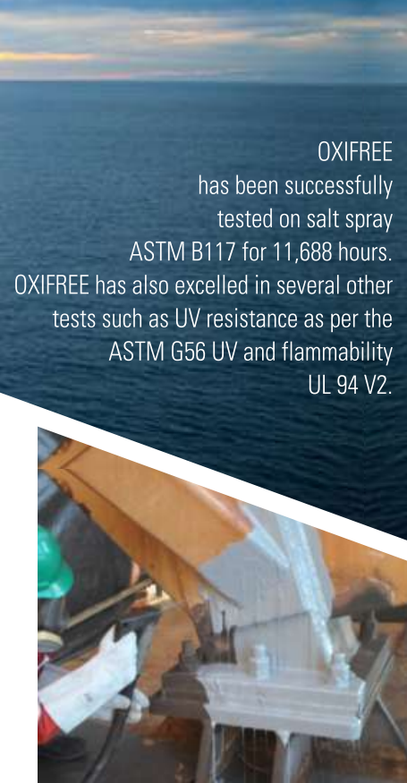
OFFSHORE PROJECT AT FPSO Foundation of hose reel aft offloading
